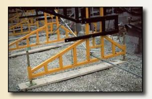
**BASE UNIT** - The 7' wide steel base is 2' high and provides system stability. Included with the base unit are large diameter leveling jacks. Horizontal braces are used to connect base units together and assist in squaring freestanding tower sections during set up and use.
