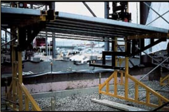
**TENDER BRACKET / MASON BRACKET** - The tender bracket carries a 4,000 lbs. rated capacity with a 4:1 safety factor as required by OSHA Regulations (independent laboratory tested). This bracket can accommodate either 4 or 5 wood or metal boards. The mason bracket provides a large platform area that accommodates either 2 or 3 wood or metal boards. A complete guard rail and toeboard system is included with the Mason-Jax Scaffold System.
