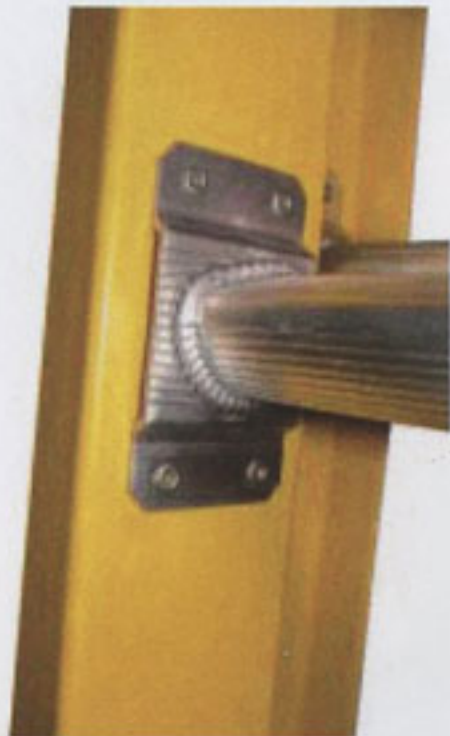
Plate to Rail Rung Connection
